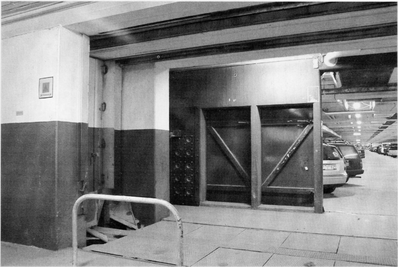
Stockholm Civil Defence Shelter - Blast doors. Photo Dan McKenzie
